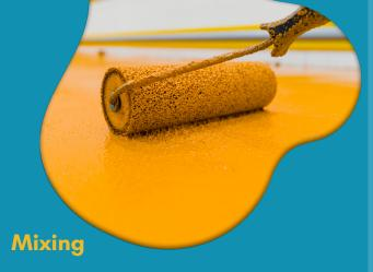
Part A Polyol should be shaken before being poured into the barrel. Next, add all of Part B and Part A to the clean mixing barrel and mix for 5 seconds with a 750-watt high-power mixer. After that, add only the pigmented Part C mix for 5 seconds, and finally add only the Part D powder. Mix for at least 20 seconds to achieve a homogenous consistency.
